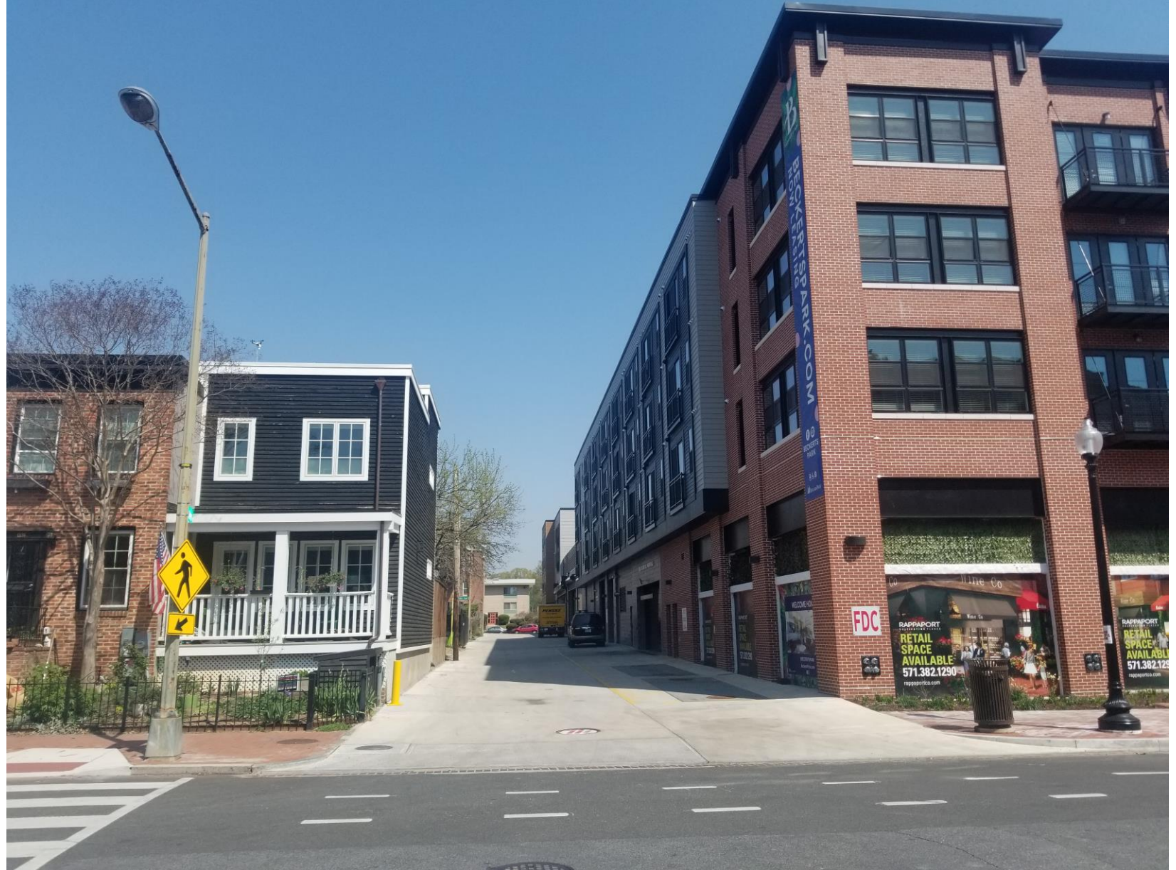
Similar Building: 35' of Separation
